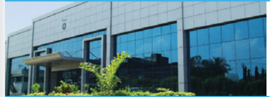
State-of-the-art Solid Dosage & Lozenges manufacturing facility at Kadaiya, Daman
