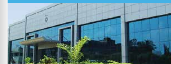
State-of-the-art Solid Dosage & Lozenges manufacturing facility at Kadaiya, Daman
