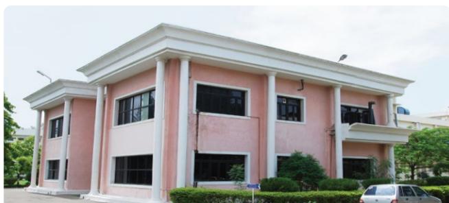
State-of-the-art US FDA approved API facility at Panoli, Gujarat
