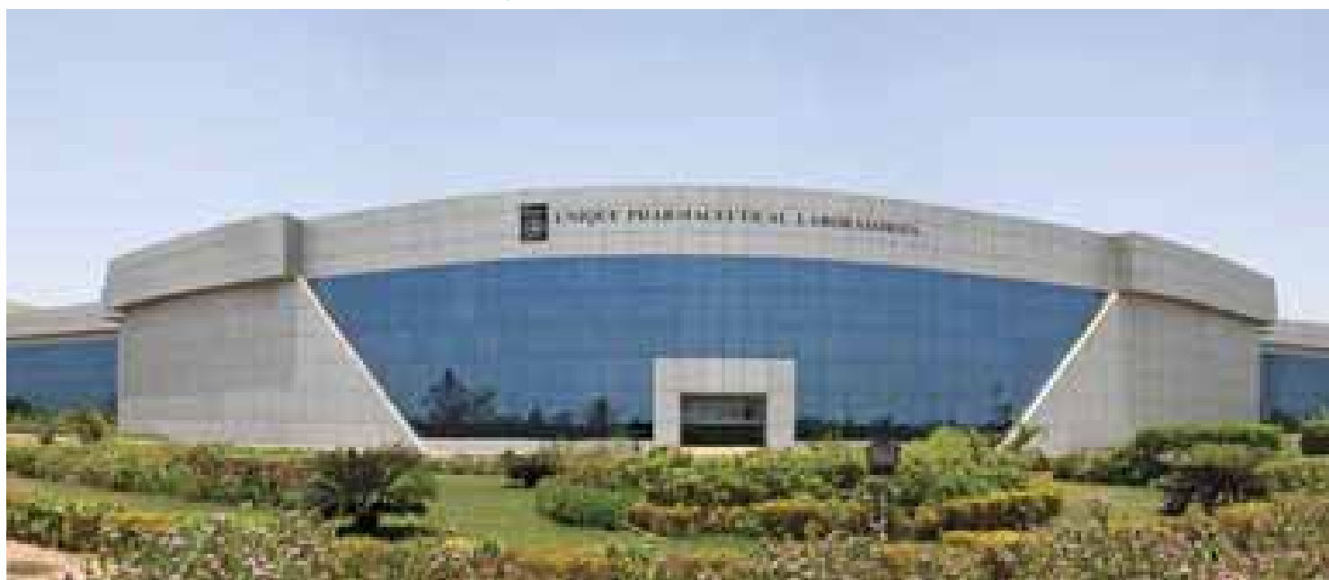
State-of-the-art Formulations manufacturing facility at Panoli, Gujarat
