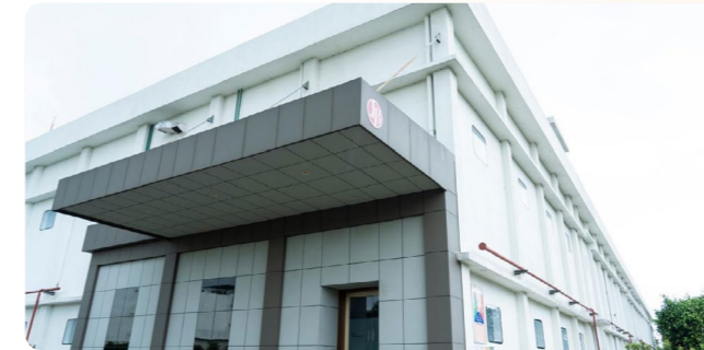
State-of-the-art T20 US FDA-accredited solid dosage manufacturing facility at Panoli, Gujarat
